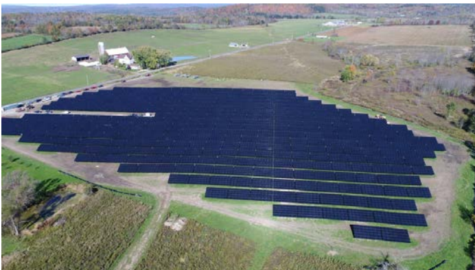
2.0 MW CIGS (Left) and c-Si (Right) PV installations in Oppenheim, NY.
