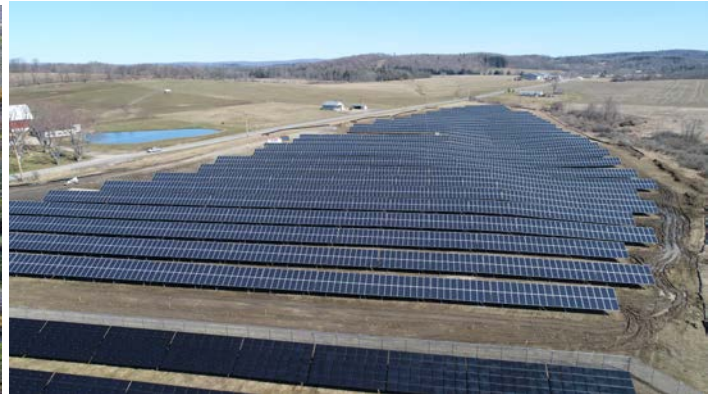
2.0 MW CIGS (Left) and c-Si (Right) PV installations in Oppenheim, NY.
